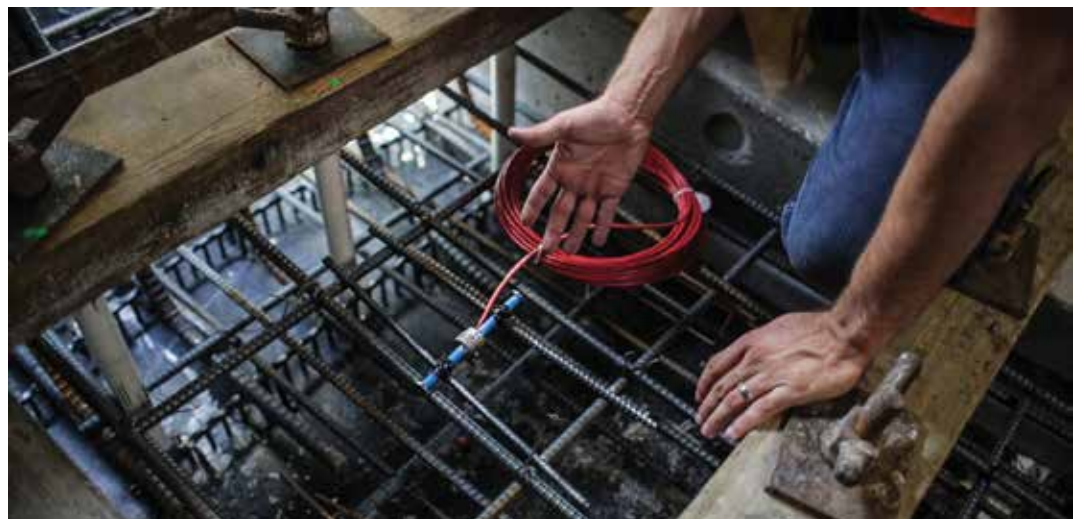
Figure 3: Image of FIU engineers installing 96 sensors in critical locations on their new flyover bridge
