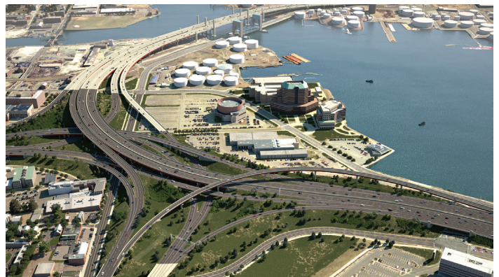
Figure 1: Reality Computing enables the direct capture of spatial information about the real world, use of that data in design processes, and delivery back to the physical world. Reality Computing technologies were used to carry out the I-95 New Haven (Connecticut) Harbor Crossing Corridor Improvement Program, pictured here in a digital rendering of the proposed infrastructure improvements. Image courtesy of Parsons Brinckerhoff
