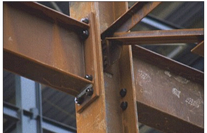
Figure 2: Typical beam to column connection.
